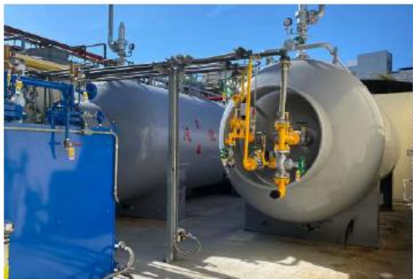
Switching steam boiler fuel from heavy oil to LPG
