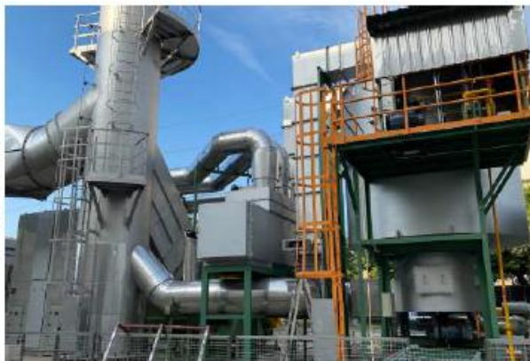
Zeolite rotor concentrator & regenerative thermal oxidizer (RRTO) for VOCs
